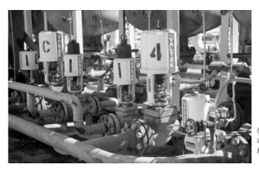
(right) A liquid nitrogen loading facility in Australia uses two Mark One valves for its emergency fire water system.
