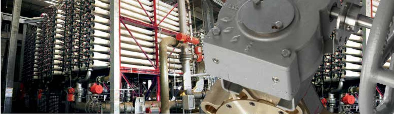
**SEA WATER:** Bray/McCannalok valves have been successfully installed in power plants, desalination plants and offshore drilling projects. Duplex, super duplex and super austenitic stainless trims can be provided for sea water service. Higher alloy materials are available.
